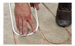
Starting from the manifold and following the Inva-Heat design, loop the pipework into the channels of the chipboard in a serpentine pattern and return back to the manifold or to the point the 12mm pipe connects to the flow and return.
