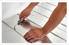
Install the pipework by pressing it firmly into the grooves. Where the pipework is connected to the manifold there will be a need to use plain insulation and clips to take into account the closer pipe centres.
